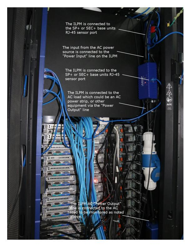
The above installation example shows how the ILPM is connected to the SP2+ unit and the AC equipment installed in this server cabinet.
